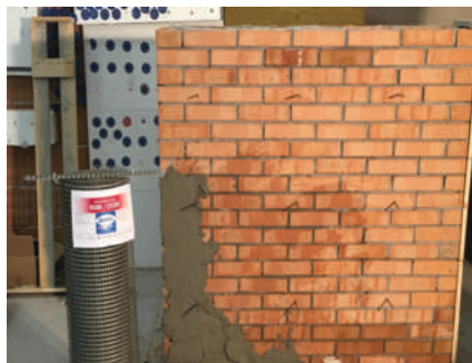
2. PRIMA MANA DE MORTAR STRUCTURAL BIO FORCE ONE
